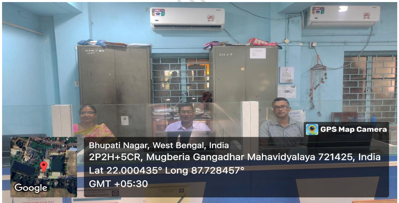
AC facility at office
